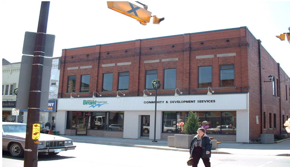
Community & Development Services Office
