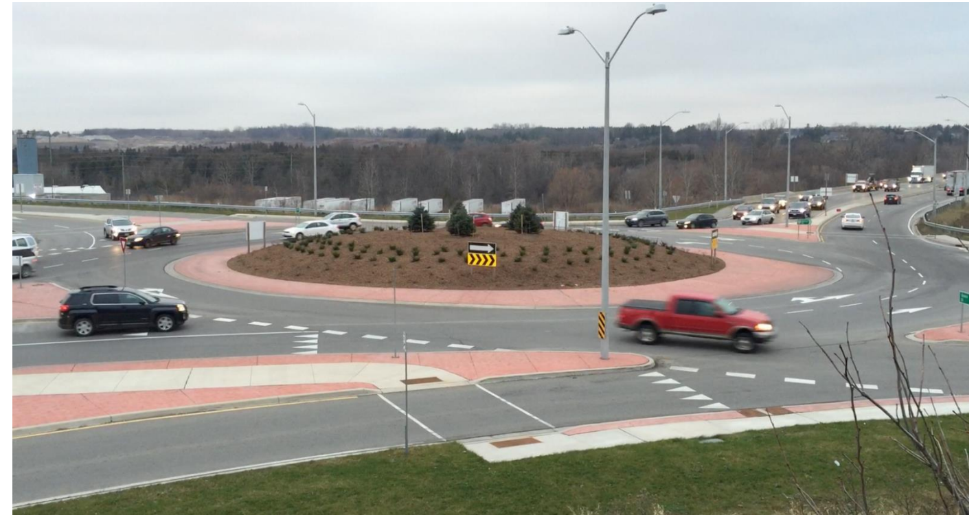
Photo 1: Example of Roundabout (Hespeler Road, Cambridge, Ontario)
