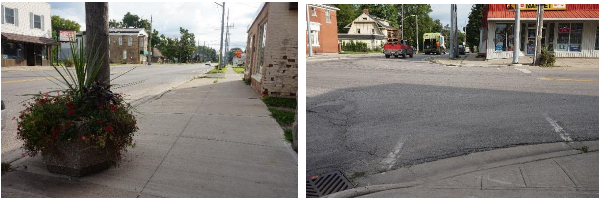
Existing sidewalks and crossings
