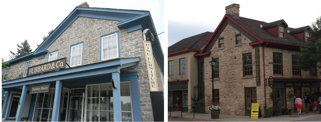
Examples of restored windows and storefront windows (examples from Spencerville, Ontario and Perth, Ontario)
