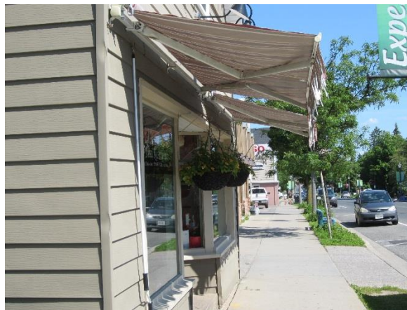
Fabric awnings which complement the façade are preferred (example from Erin, Ontario)
