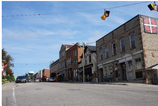
St. George has a mix of roof styles, but principally flat roofs
