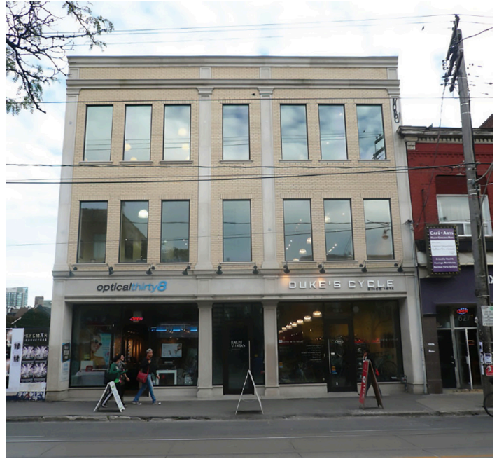
Example of a new building with clearly defined facade articulation. This can be further improved by using windows with mullions.
