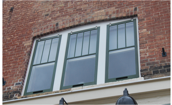
EXAMPLE OF RESTORED WINDOWS
