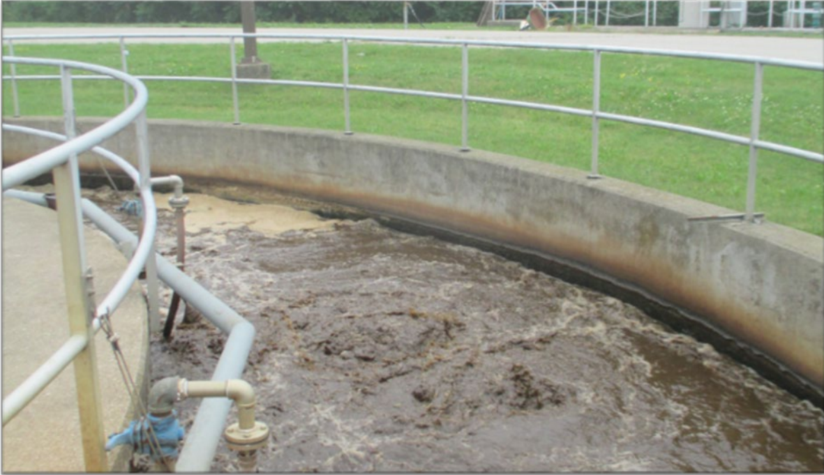
Figure 14 Aeration Tank Surface (July 2014)
